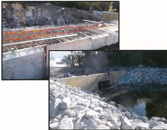
48-inch and Box Culvert Construction Rubble Rip-Rap Outfall
