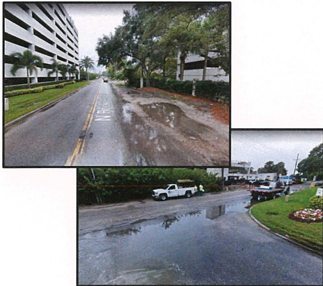
Re-profile Roadway to Alleviate Standing Water
