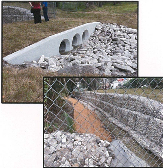
Bishop Creek Conveyance and Water Quality Improvements
