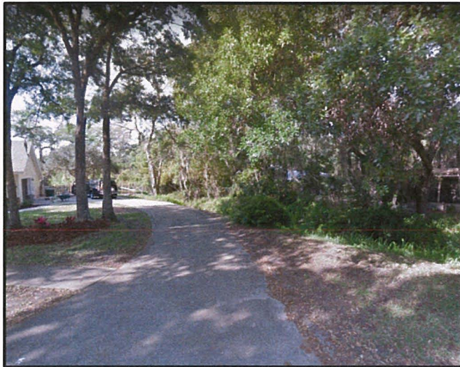
Emergency Stormwater Repair Project due to Potential Driveway Collapse
