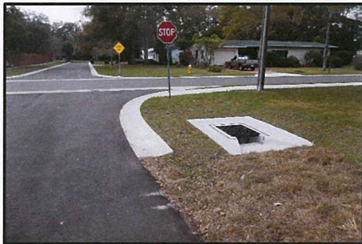
Neighborhood Street Drainage Improvements Swales, Storm Culverts & Exfiltration Trenches
